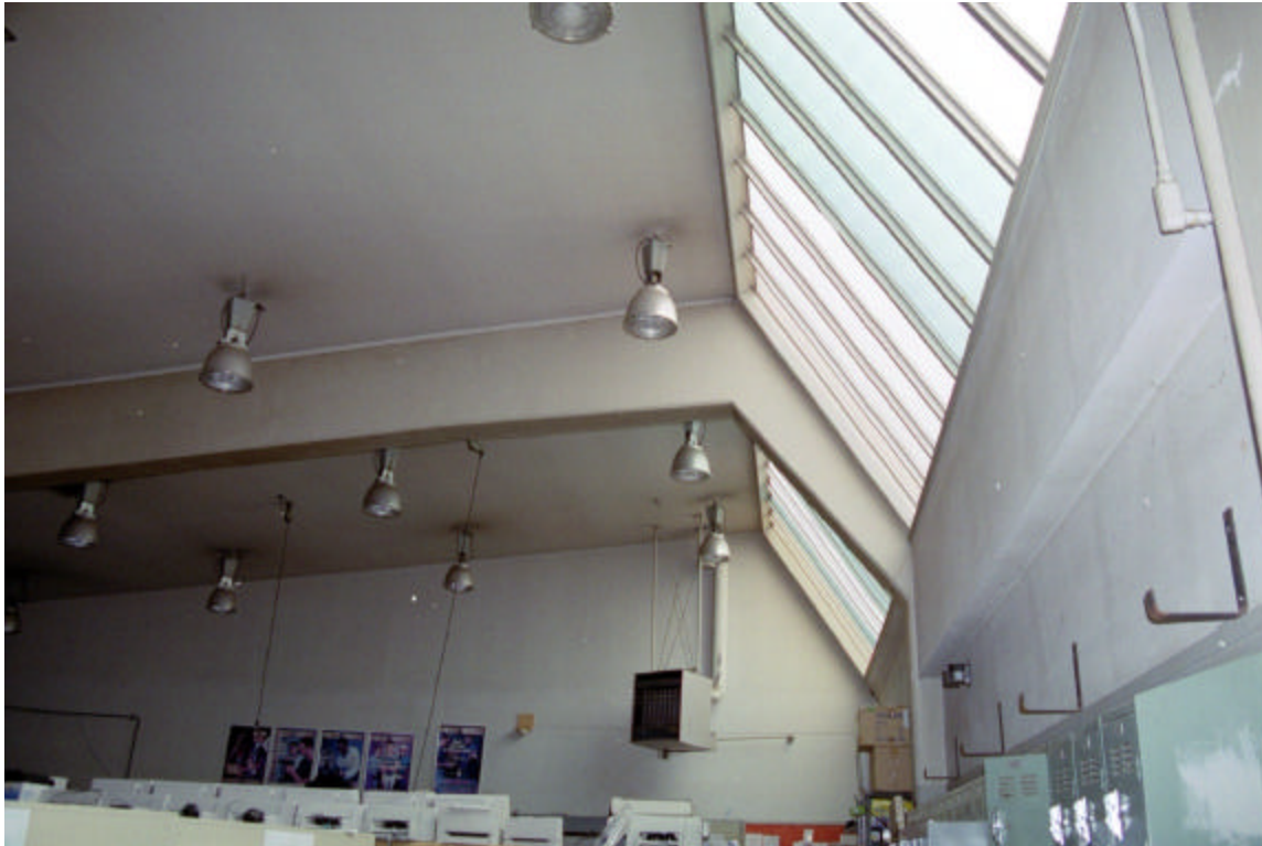
Figure 18: Interior of the industrial arts building
