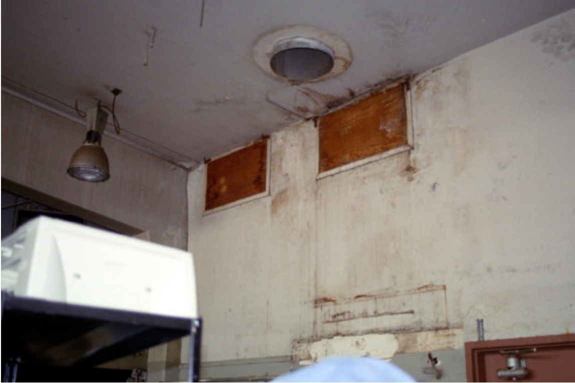
Figure 20: Deterioration of the wall in the industrial arts building
