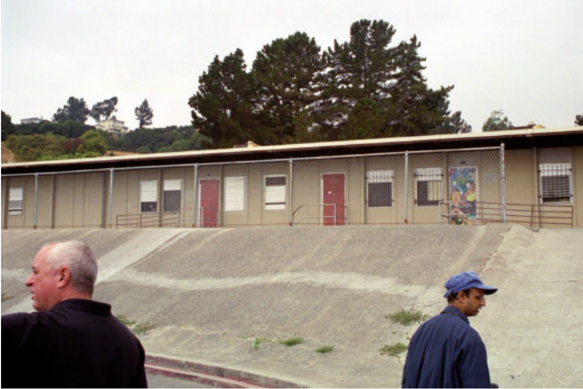
Figure 22: Portable classroom units
