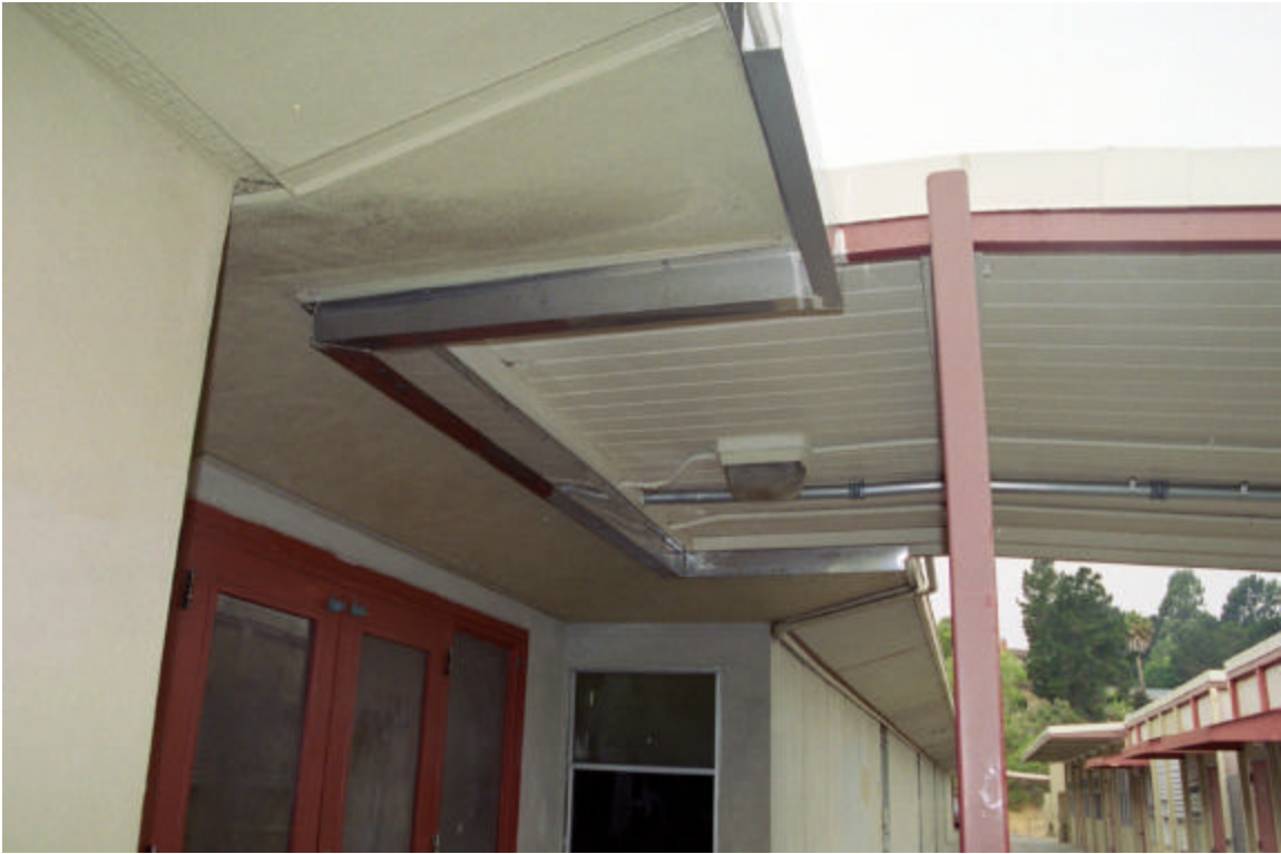
Figure 9: Setback in roof of the classroom building at the entrance
