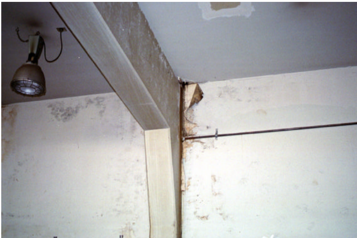
Figure 19: Deterioration of the wall in the industrial arts building
