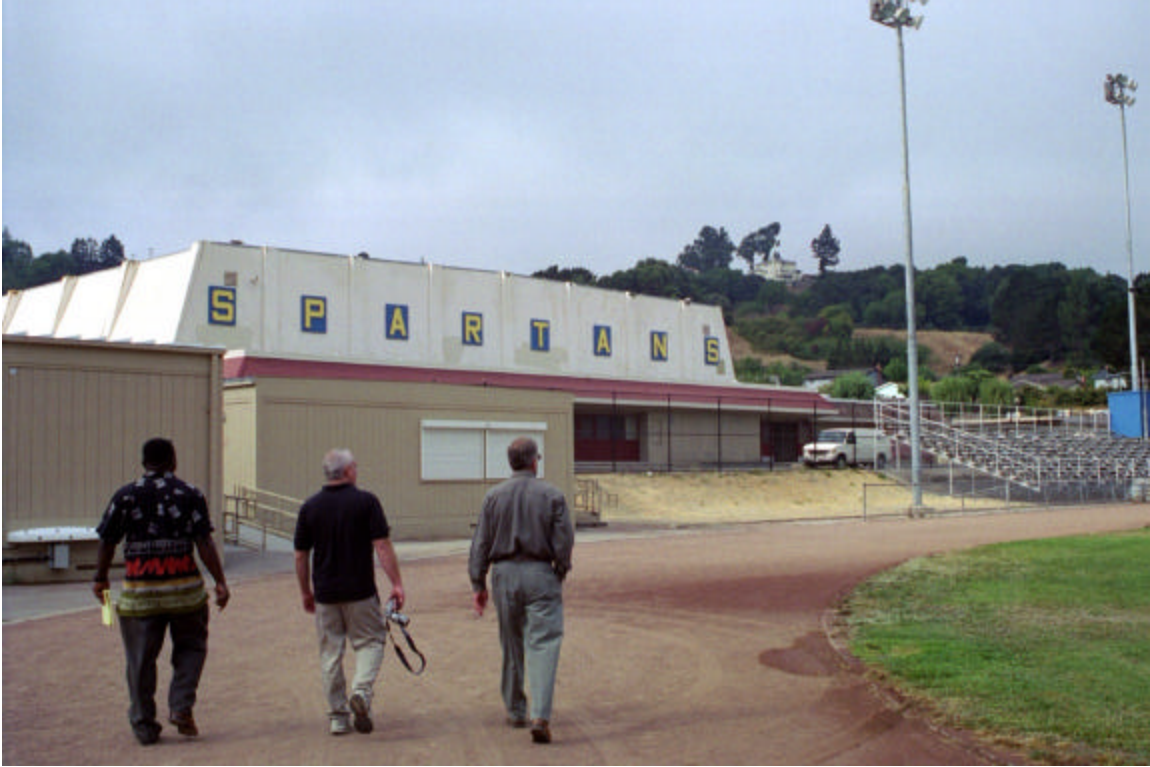
Figure 14: North side of the gymnasium
