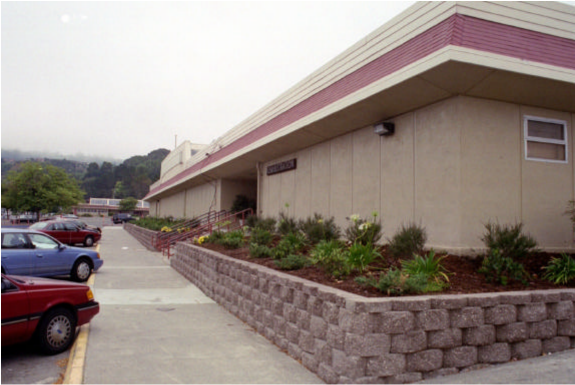
Figure 4: Northeast corner of the administration and library building
