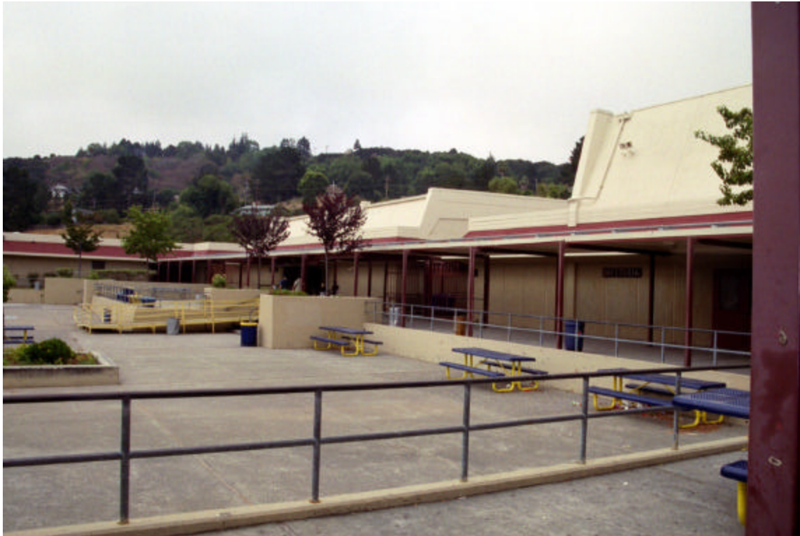
Figure 10: Front of the cafetorium and the performing arts building
