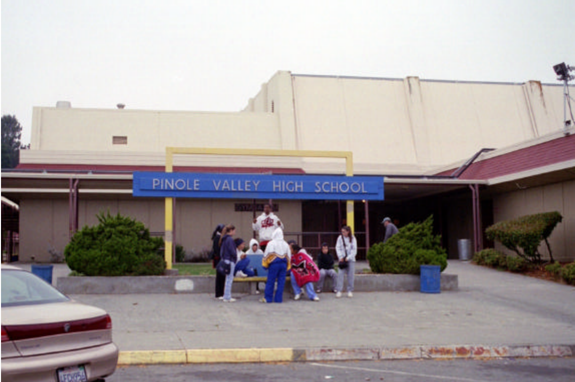
Figure 13: East side of the gymnasium
